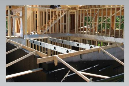
TUFF BEAM ™, TUFF JOIST™, and TUFF JOIST+™ make up the TUFF Floor™ Systems, offering the design flexibility to achieve conventional or radical floor designs. Pre-punched reinforced access holes allow plumbing, HVAC, electrical, and other technology services to be installed within the floor system to improve ease of installation while maintaining structural integrity.
